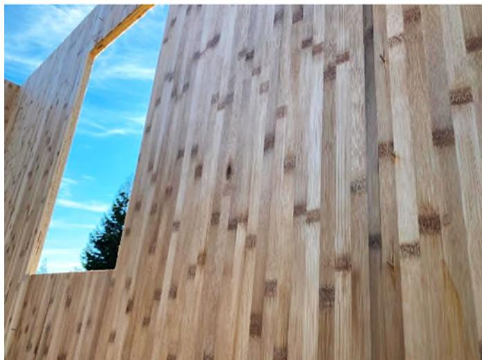
**Figure 2.** BamCore panelized Prime Wall™ system
