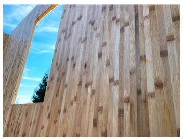
Figure 2. BamCore panelized Prime Wall<sup>™</sup> system
