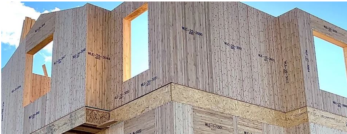
Figure 1. House Under Construction Using BamCore Prime Wall System
